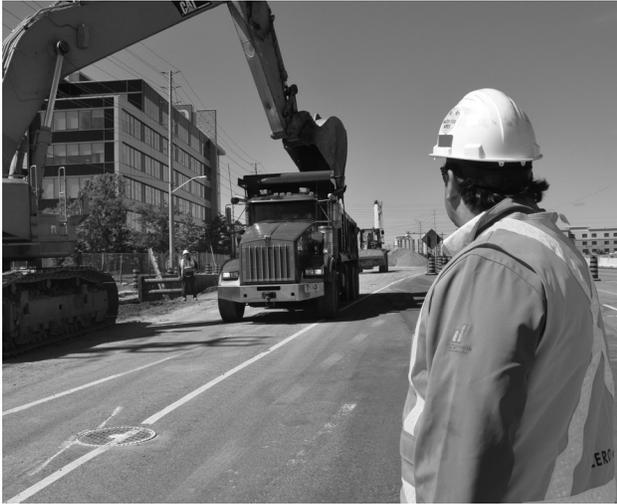
**Figure 17-1: High-visibility Clothing Helps Equipment Operators See Workers**
