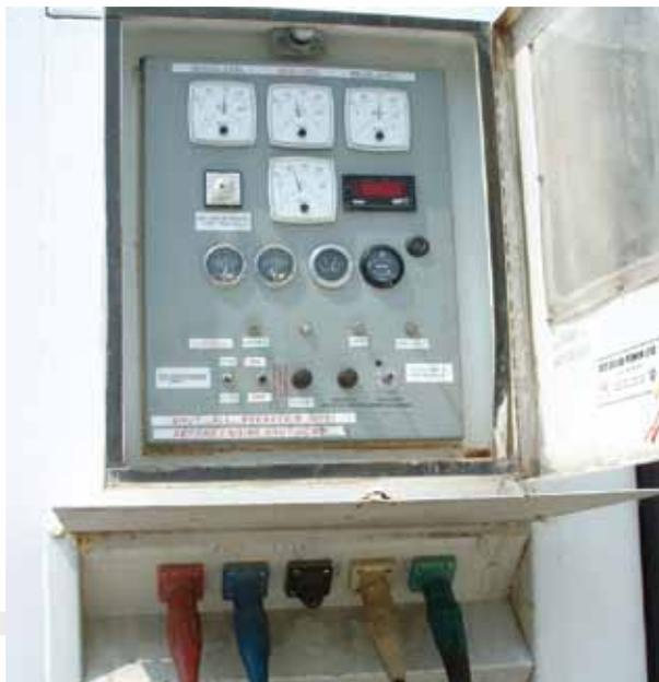
**Generators connected to Cam-Lok connectors must be inspected by the ESA**
