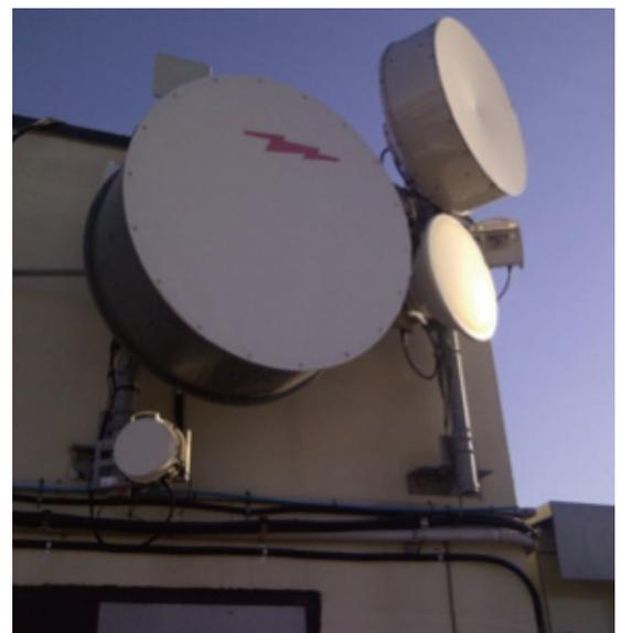
Figure 2: Drum-type Cell Antennas
