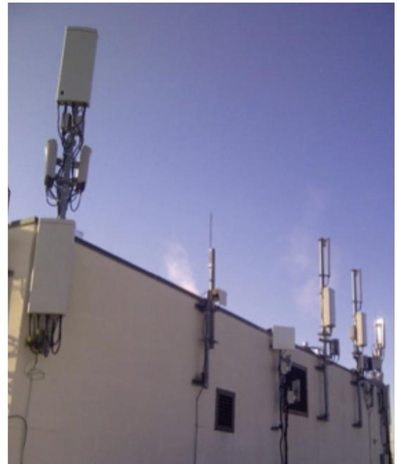
Figure 1: Paddle-type Microwave Antennas
