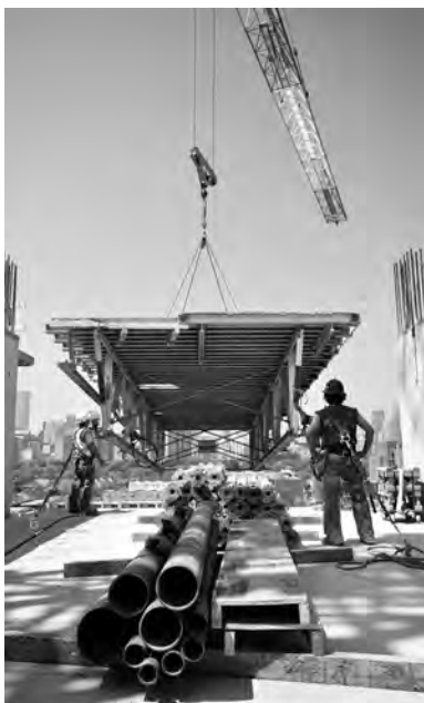
Figure 42-24: Fall Protection Required when Receiving a Flying Form
