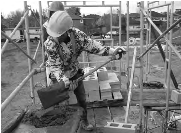
Figure 16-1: Wearing Gloves and Covering Exposed Skin Can Protect Against Hazards
