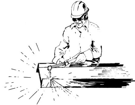
**Figure 11-15: Protection from Injurious Radiation (Gas Cutting)**
