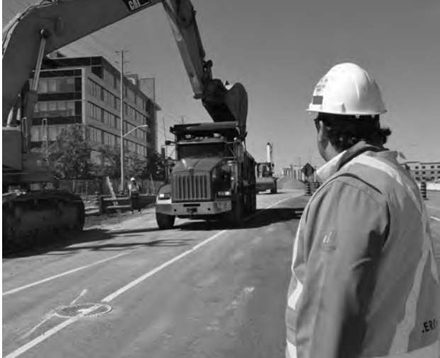
Figure 17-1: High-visibility Clothing Helps Equipment Operators See Workers
