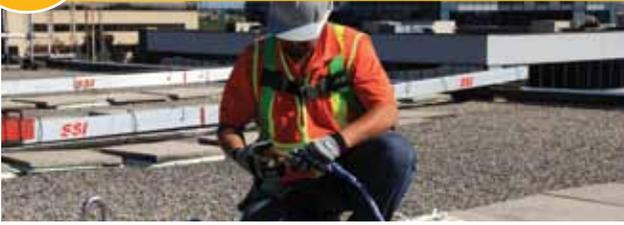
Falls are the main cause of critical injuries and deaths for Ontario construction workers.\* All workers who are exposed to fall hazards must be protected (O. Reg. 213/91, s. 26). The best protection is a guardrail system. If this is not practical, then a fall protection system must be used.
