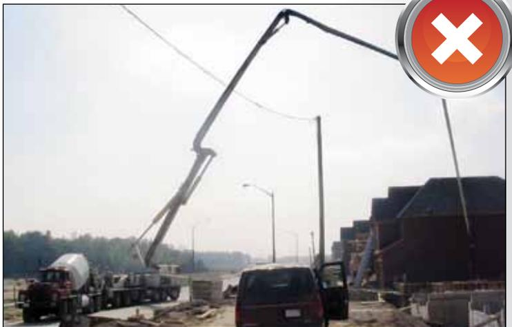
**Never extend a boom over electrical wires, even if you can maintain a safe minimum distance.**
