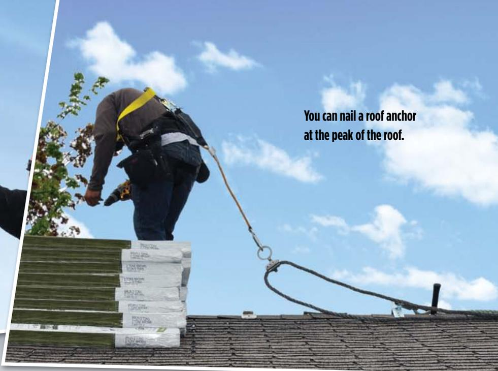
You can nail a roof anchor at the peak of the roof.
